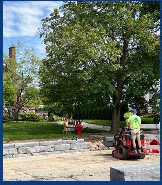
Progress continues on the Penniman wall. Most of the stone has been installed with some smaller pieces still left to finish. Next steps will include some sections of sidewalk replacement, backfill/topsoil between the sidewalk and the wall, installation of trees, shrubs, and mulch.
