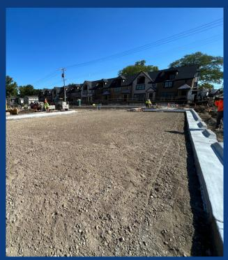
The Saxtons public parking lot is taking shape. The underground storm sewer system and storm water detention have been completed. The concrete curbs were poured and crews are working to grade the stone base throughout the parking area. Once the concrete has cured, crews will return to install the drive approaches, sidewalks and asphalt pavement.
